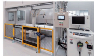
Installation of robots, paint booth, conveyor and oven.
